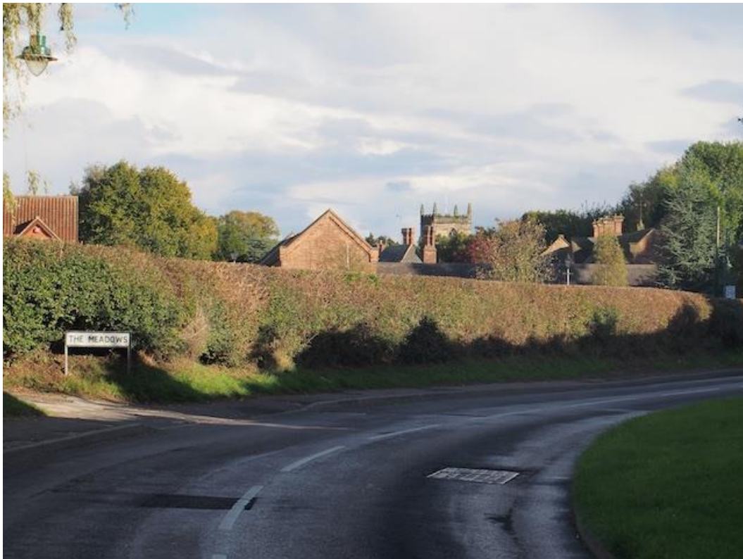
Figure 13: The view of the church tower over Taylor's Croft from Main Street
