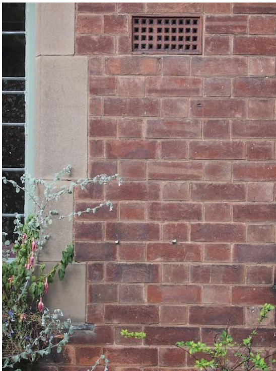
Figure 24: Flemish bond at the Four Bells
