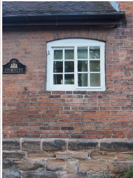
Figure 25: Yorkshire sliding sash at The Chimneys
