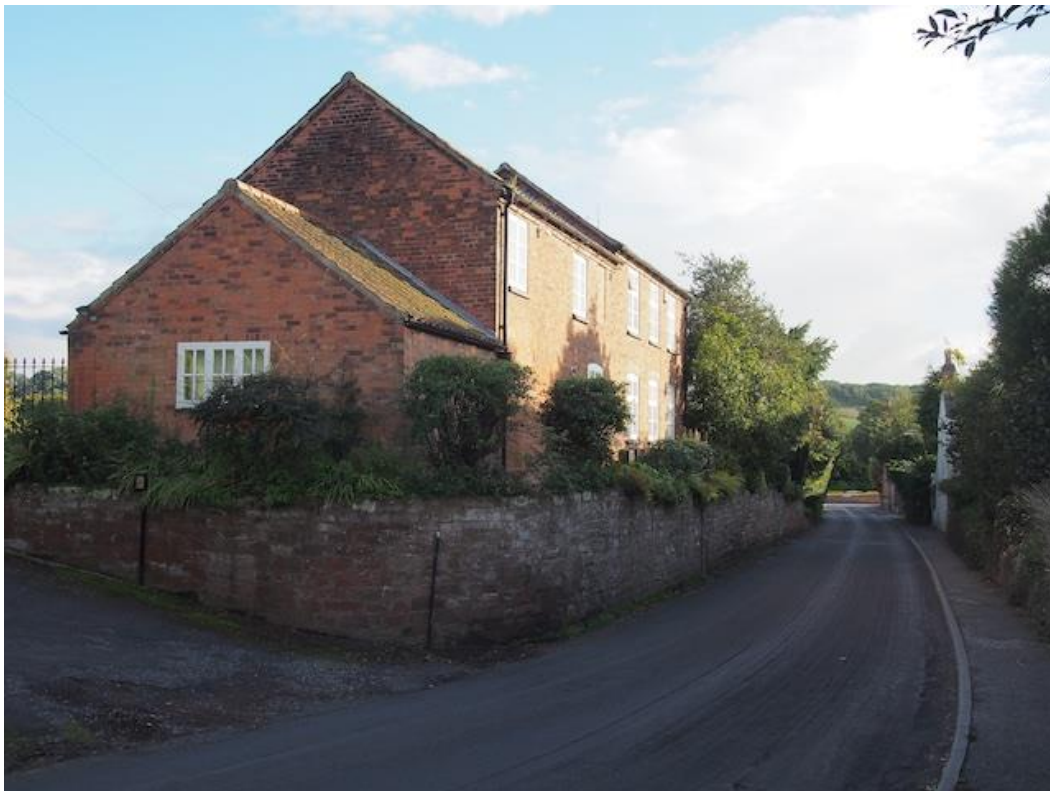
Figure 12: View south along Shelt Hill from the former Desborough factory towards its junction with Main Street, with views across the Nags Head car park
